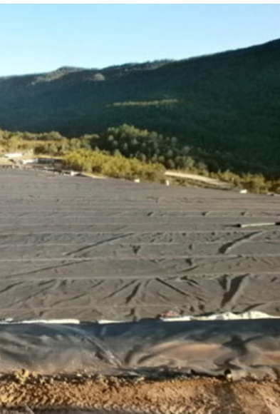
Final status of the temporary waterproofing work.
